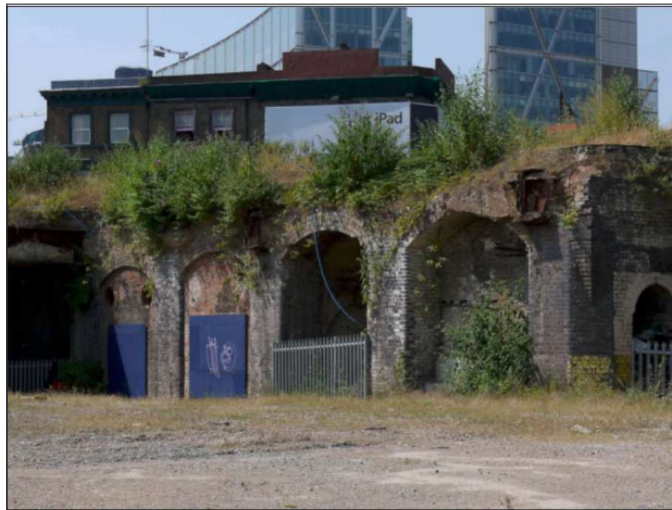
RETAINING WALL ABSENT ABOVE ARCHES ON THE EAST ELEVATION
