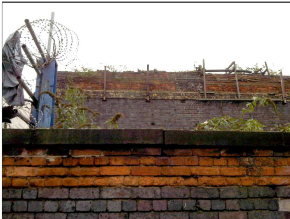
PARTIALLY COLLAPSED BRICK PARAPET TO NORTH END OF THE WEST ELEVATION
